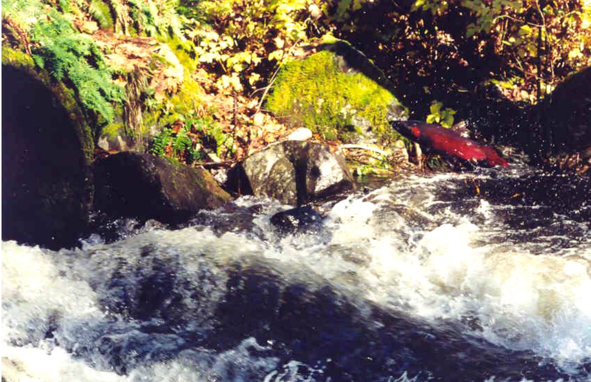
Figure 3. Coho salmon attempting to pass through a culvert at the U.S. Navy railroad bridge on Sherwood Creek (RM 6.8). The undersized culverts caused high water velocities, limiting passage of adults upstream. Photo courtesy of Allyn Salmon Enhancement Group.
