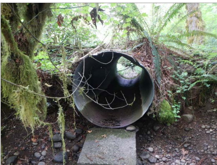
Barrier culvert winter 2013. Culvert was undersized and "perched," which prevented fish from being migrating to habitat upstream.
