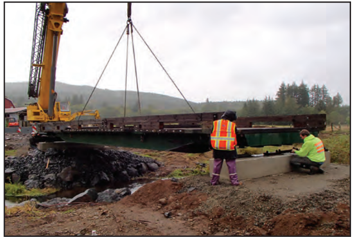
Construction team placing bridge over Gosnell Creek.
