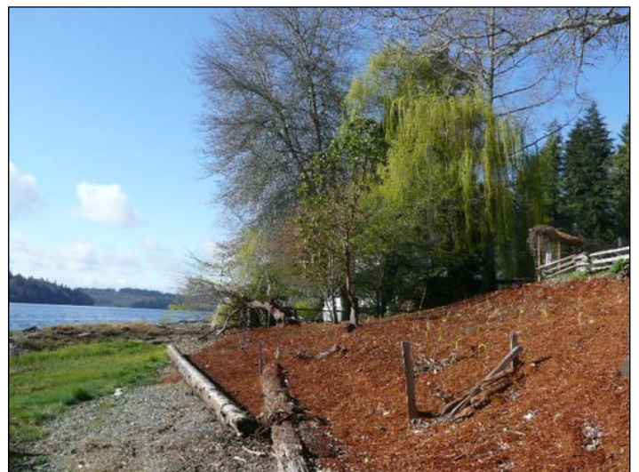
IN PROCESS: Wood chip mulch installed after ivy removal.
