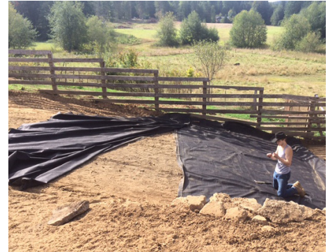
Lay Geotextile fabric
