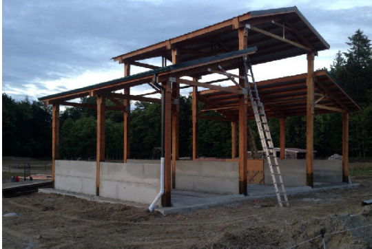
Robertson Waste Storage Structure
